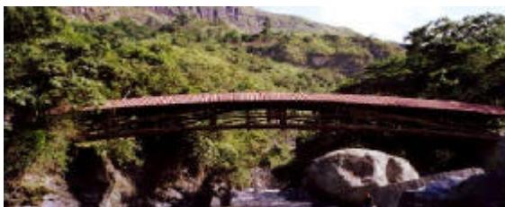
Covered bridge from Jörg Stamm
