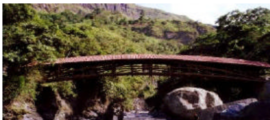
Covered bridge by Jörg Stamm
