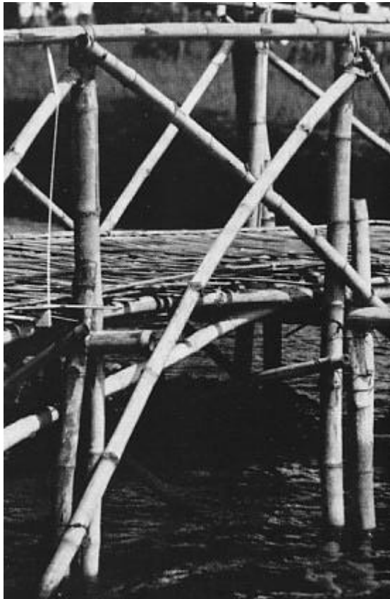
Bamboo bridge with intermediate posts
