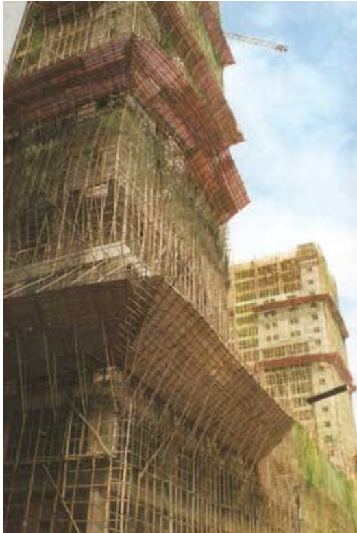
Bamboo canes used for scaffoldings
