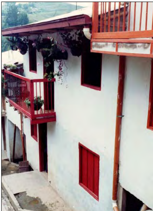
Two storey houses of bamboo construction with lime-cement plastered walls on sloped terrain. In this design low-angle fibre cement roofing has been used.
