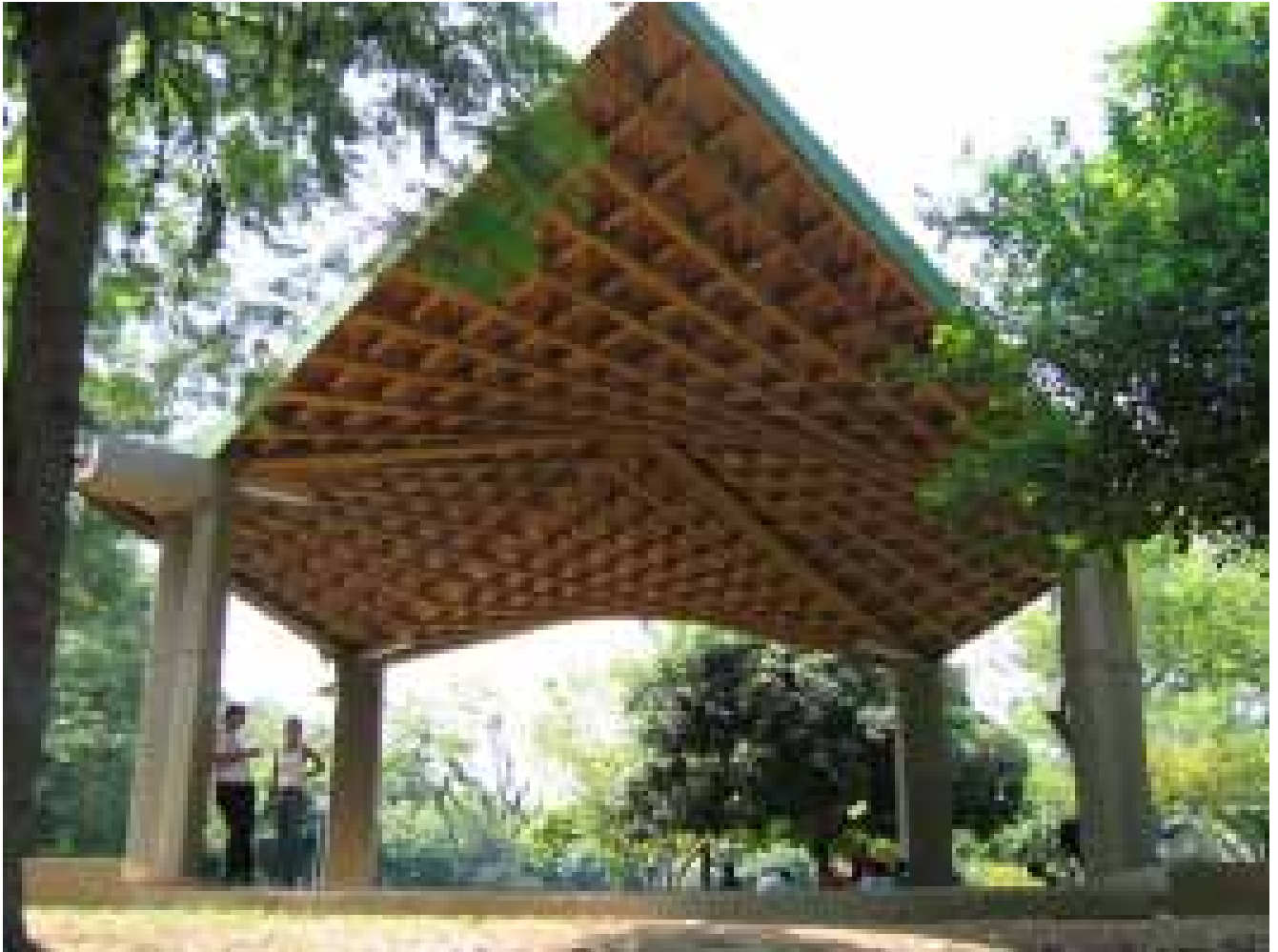
Hyperbolic paraboloid in a Colombian public park by Rafael Rojas and Hector Fabio Silva
