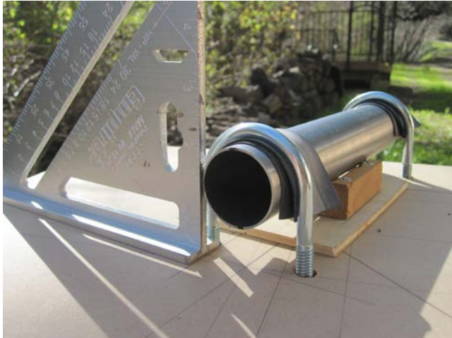
Figure 18. Using a carpenter's square and carefully marked lines on the MDF to position the head tube.
