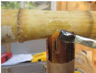
Figure 11. Applying epoxy resin to a pre-tacked joint.
