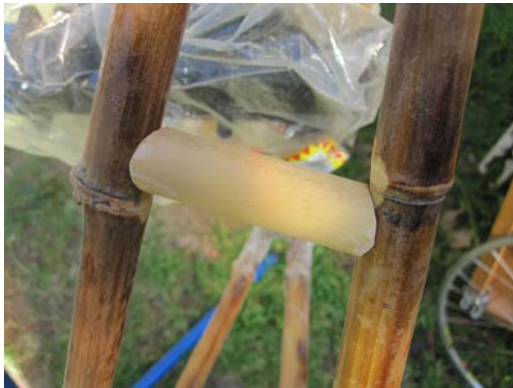
Figure 24. Initial mitering of upper cross brace.
