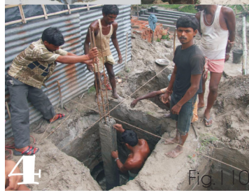
Excavate pit for foundation
