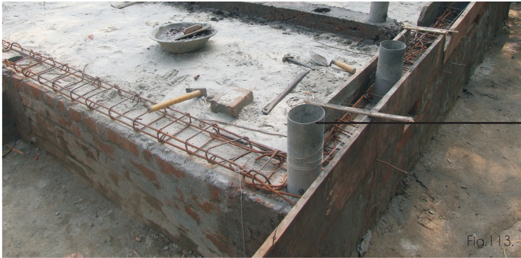
PVC Pie place in Plinth Reinforcement
