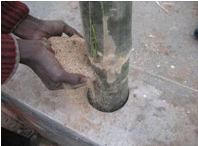
Fig.52. Bamboo Fixing at Plinth level
