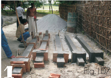
Fixing of pile in foundation
