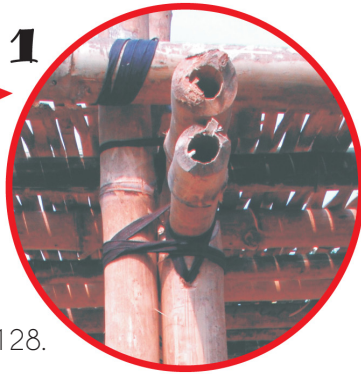
Joint at attic corner
