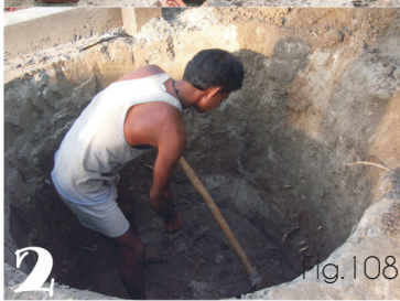
Excavate pit for foundation
