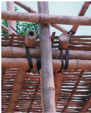
Join middle column with attic
