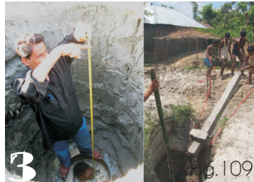
Fixing of pile in foundation
