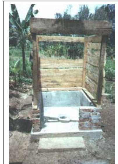
Figure 16: Toilet (under construction), directly connected to the plant Photo: Kellner (TBW)
