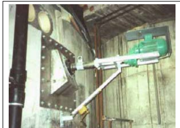
Figure 19: Stirring device for a european biodigester
