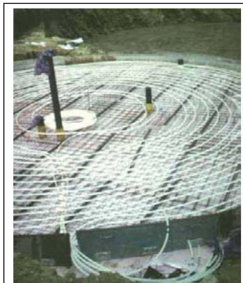
Figure 31: Heating system for a biogas digester under construction (Germany)
