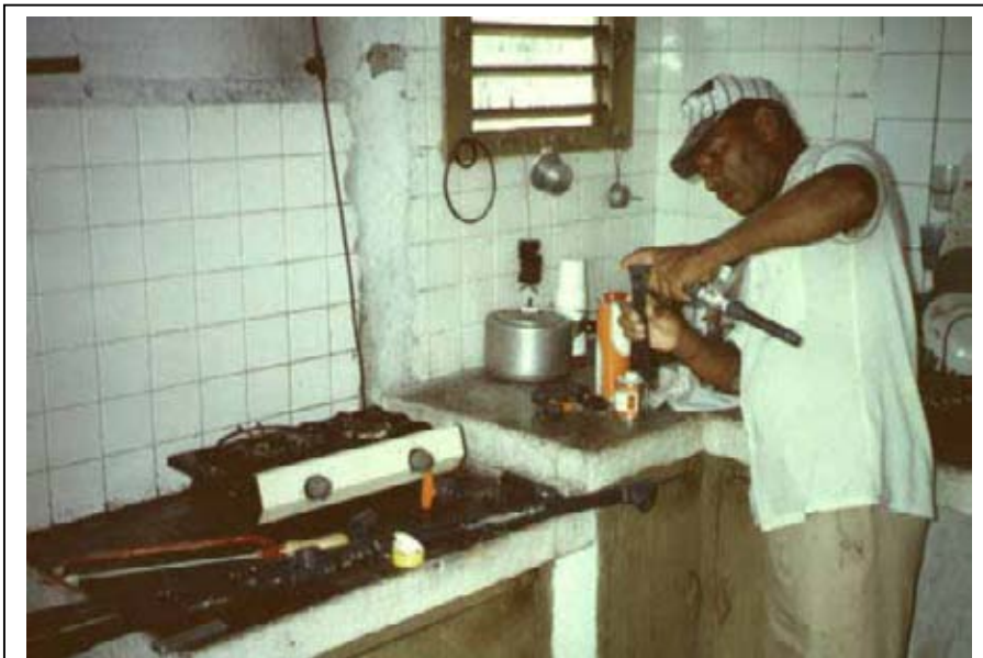
Figure 26: Final touches on a piping system with PVC pipes Photo: Krämer (TBW)
