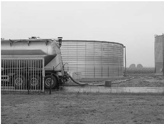
Figure 4.51 Storage tank and transportation of residue. 91)
