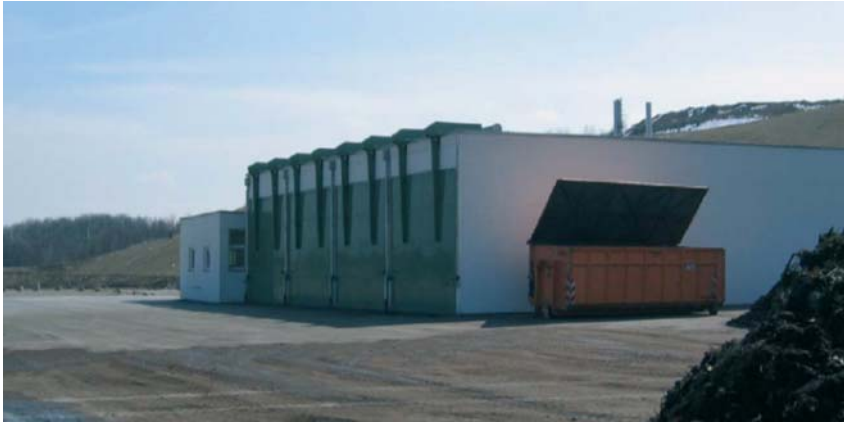
Figure 4.48 Four big size bioreactors for batch dry fermentation. 87)
