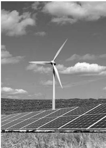
Figure 5.1 Wind-driven generator, photovoltaic and energy crops.
