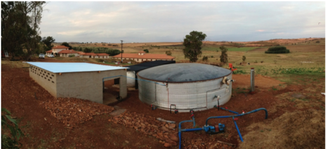
Figure 1: 150 kWh plant at Caesarsvlei
